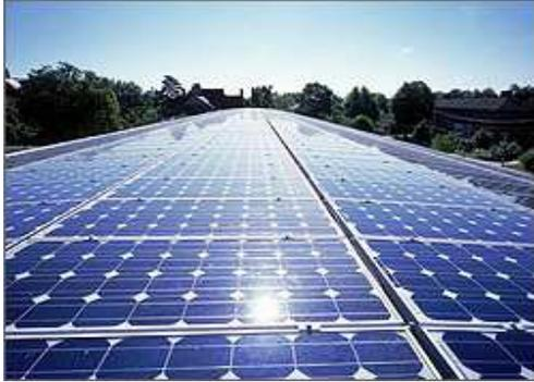
Traditional solar cells are made from silicon, are usually flat-plate, and generally are the most efficient. Second-generation solar cells are called thin-film solar cells because they are made from amorphous silicon or nonsilicon materials such as cadmium telluride. Thin film solar cells use layers of semiconductor materials only a few micrometers thick. Because of their flexibility, thin film solar cells can double as rooftop shingles and tiles, building facades, or the glazing for skylights.
