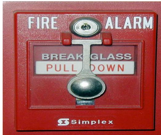
In larger buildings this may take the form of a mains operated system with break glass alarm call points, an automatic control unit and electrically operated bells or sirens.
